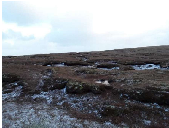
Photo 12: Erosion features at Ritten Hamar
