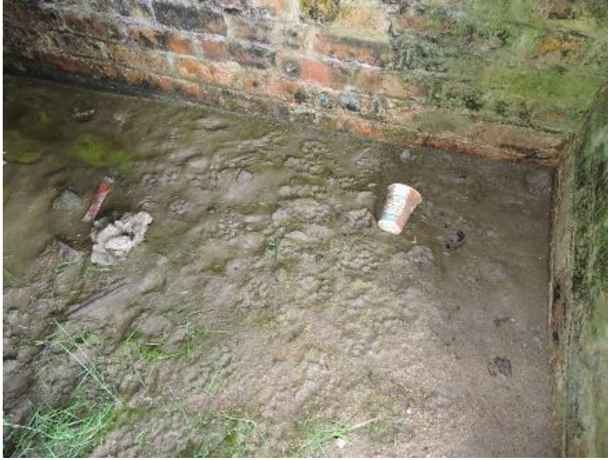
Photo 3: Fresh otter prints, of two different sizes, were clear within this abandoned military building (OS grid reference HP 67439 15637).
