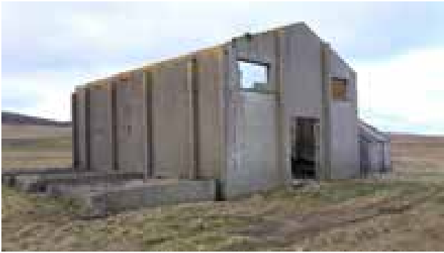
Photograph 07 – Former power station building
