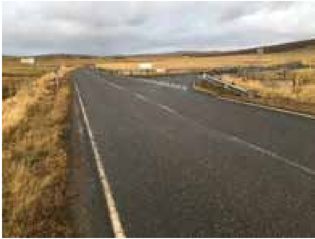
Photograph 21 Route option 1 – Junction of A968 / Beach Road
