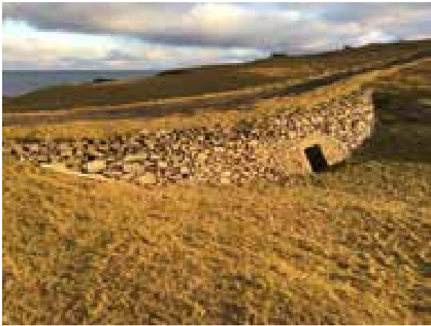
Photograph 14 – Built-up section of access track
