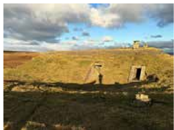
Photograph 12 – Former Transmitter Block
