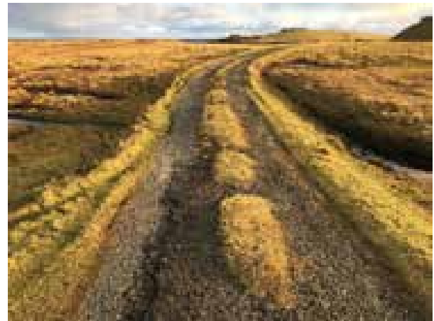
Photograph 10 – Access track looking east
