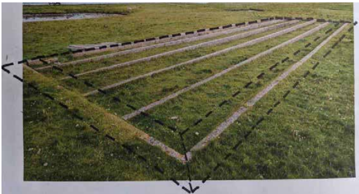
Fig. 11: Consider burying vulnerable foundations and footings. This would require accurate recording beforehand, which would allow future understanding of the site and could be used as a basis for interpretation. Final details require further discussions, however, the structure could be separated using geotextile membrane and gravel, before covering with sloping soil and grass which would allow the feature to be clearly visible.
