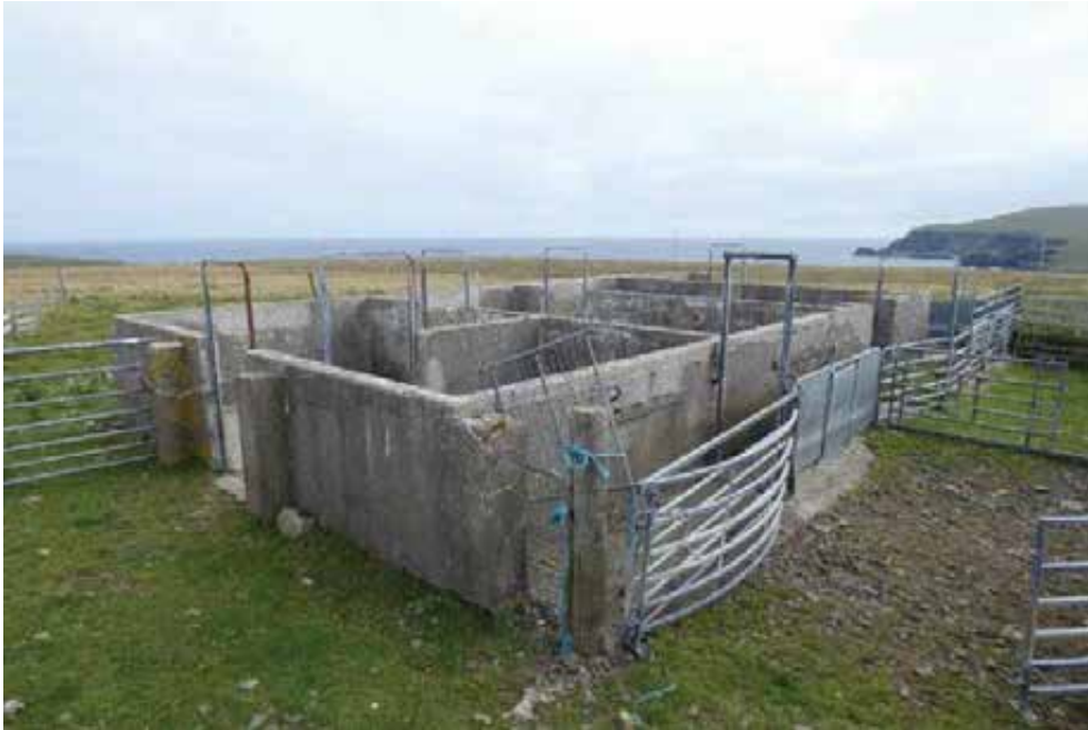
View from northwest. Walls have been lowered, with rendering patch repaired and gates inserted to accommodate agricultural use.
