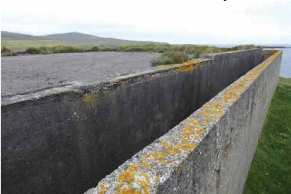
Looking across the surface of the roof. Note missing parapet copes and vegetation growing on roof.
