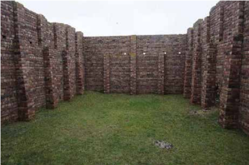
Internal general view.
