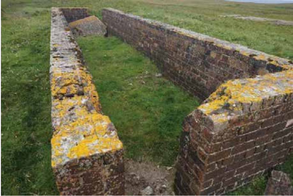
General internal view from south.
