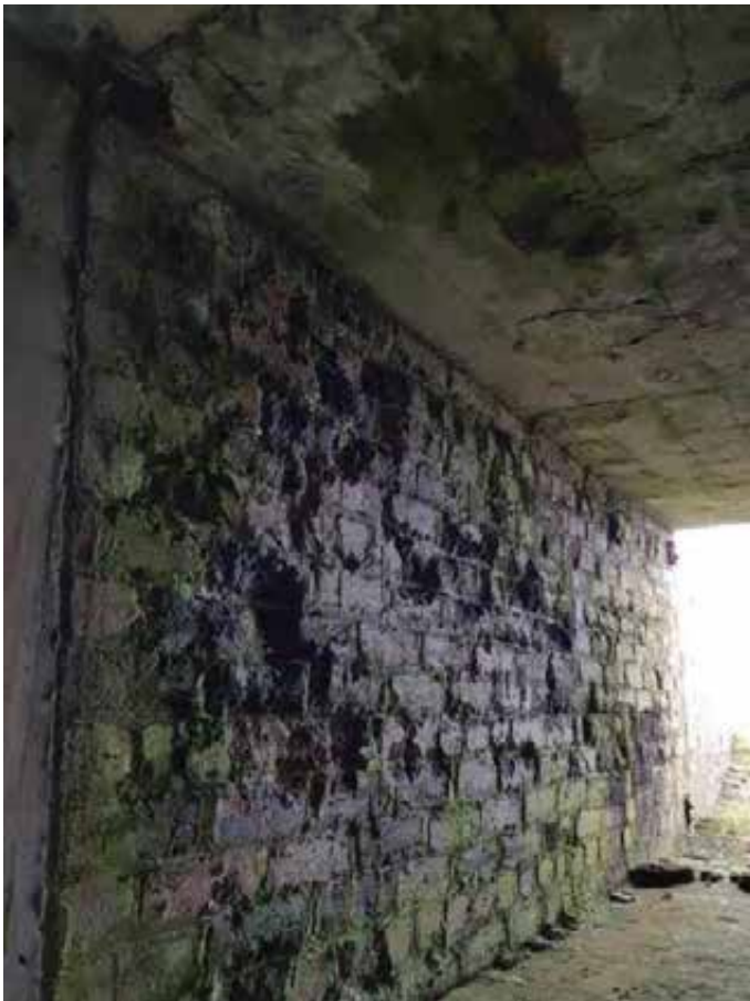
Brick wall and RC roof of duct tunnel.
