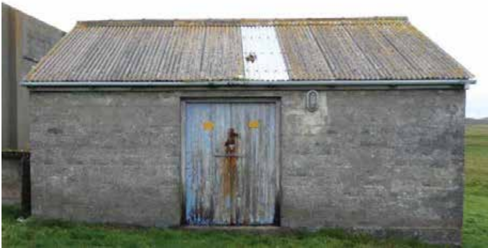
East elevation: Replace rainwater goods. Joinery repairs to doors prior to full joinery redecoration.
