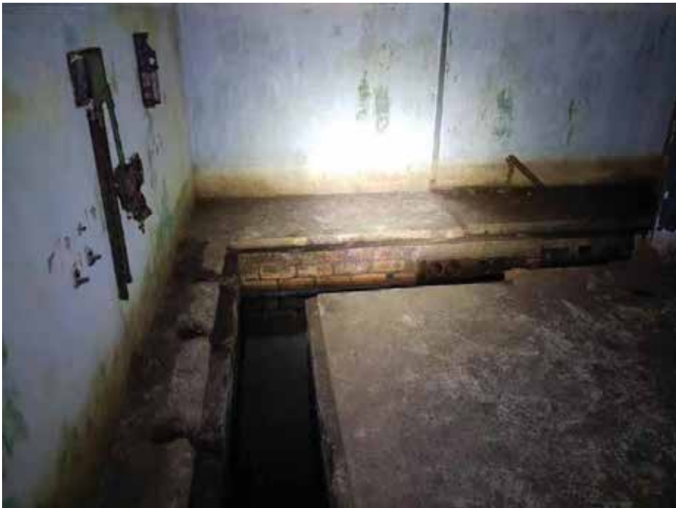
Open floor trench.
