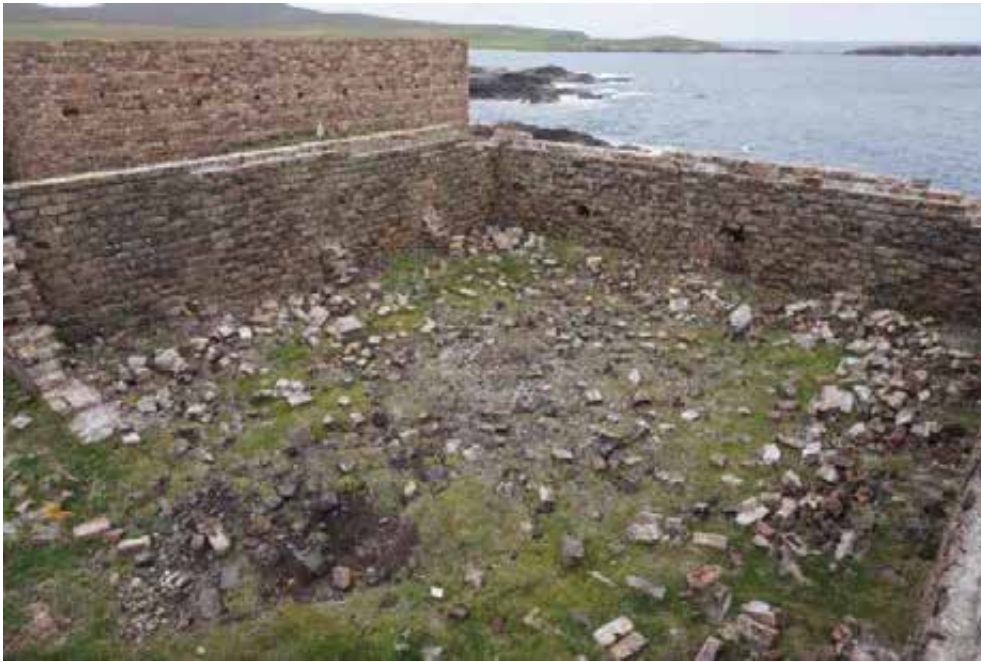
General view internally.
