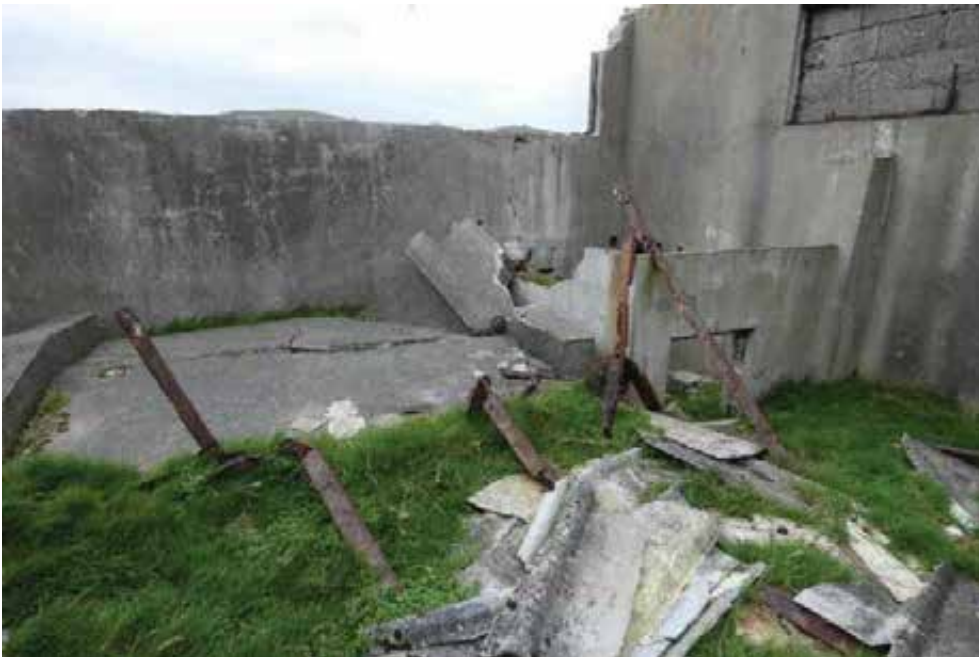
Inside of the west gable. The collapsed upper section can be seen on the floor.
