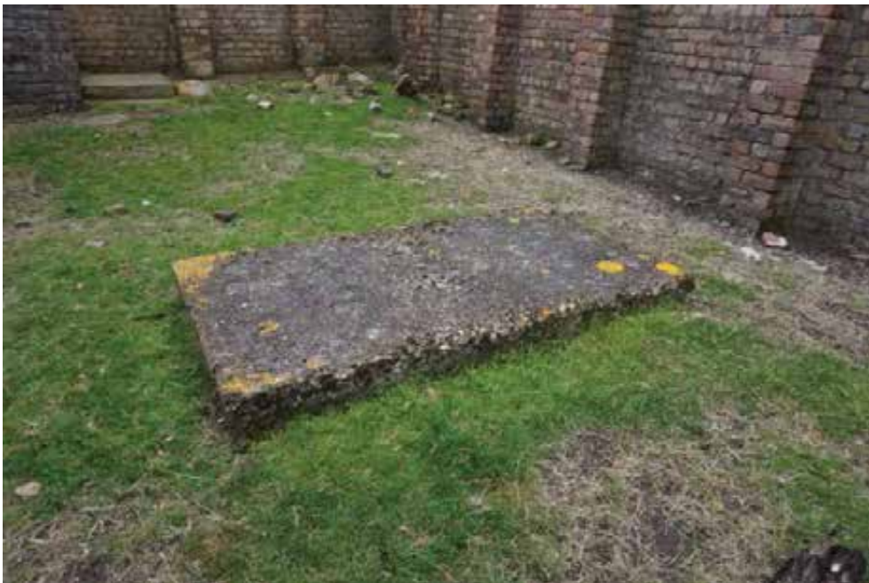
The concrete base internally is in good condition.
