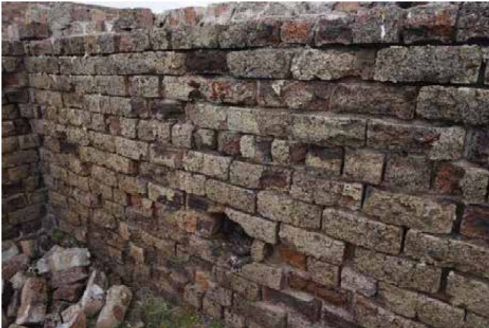
The internal faces are badly fire damaged, requiring extensive consolidation including repointing, resetting loose bricks and replacing badly damaged bricks.
