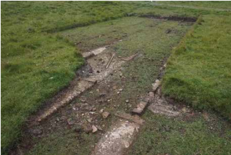
Loose brick footings, disaggregated concrete strip foundations and displaced bricks, timber and metal work at southern portion of the structure.
