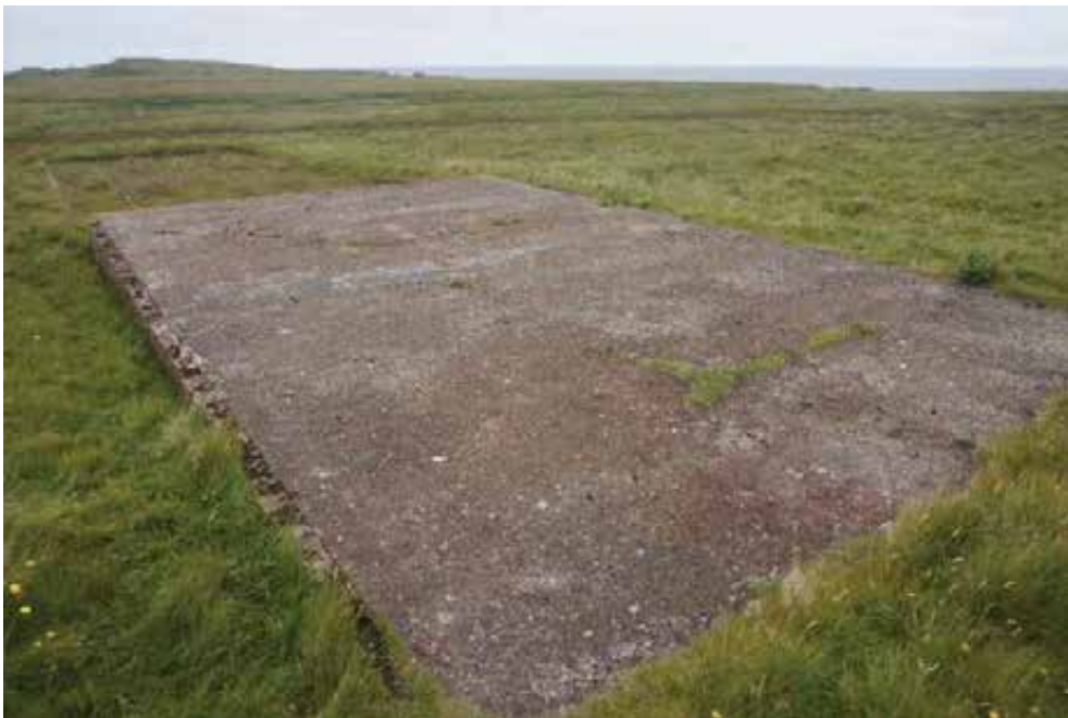
General view from northwest of west portion comprising concrete floor slab surrounded by part buried brick footings.
