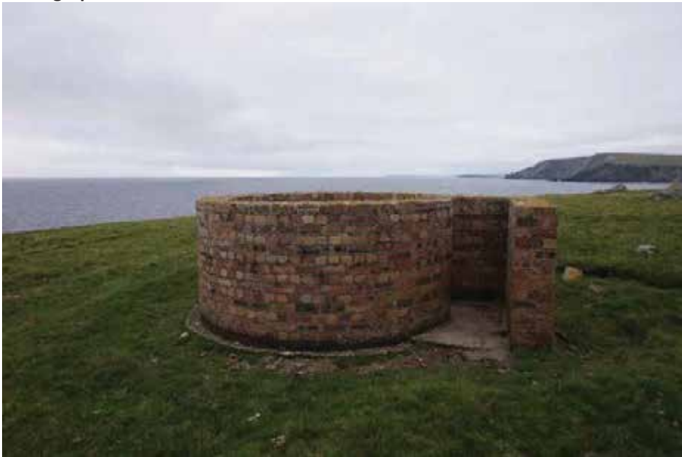
View from east showing concrete strip foundation and concrete floor.
