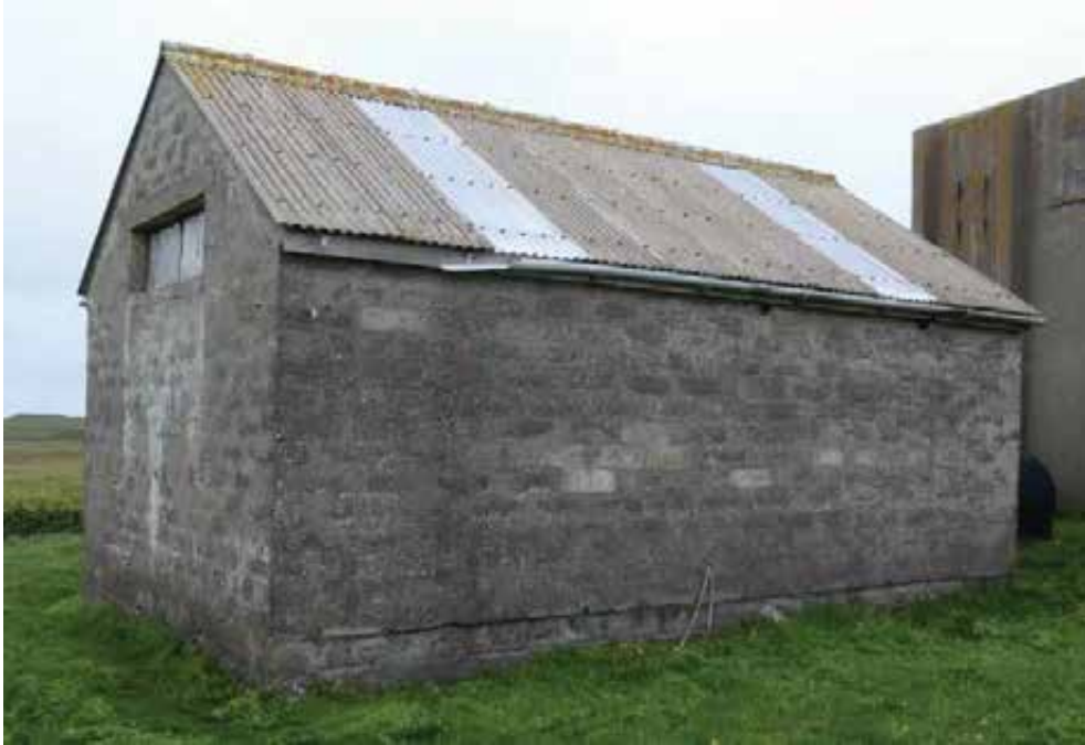
West elevation: Replace rainwater goods. Decorate facia.
