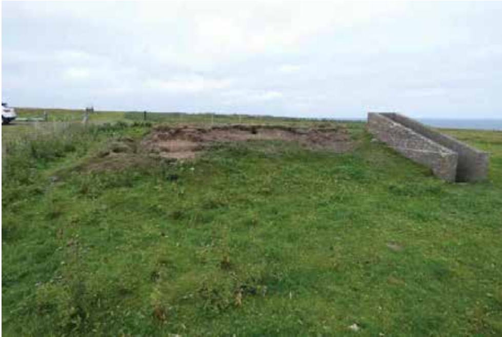
General view from southwest. Note damage caused by grazing and burrowing animals.
