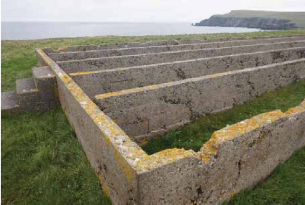
Damaged concrete is limited to the perimeter walls, suggesting it was caused during demolition works and removal of the wallplate fixings or when the fixings corroded at a later date causing localised spalling. Note poorly mixed and compacted concrete.
