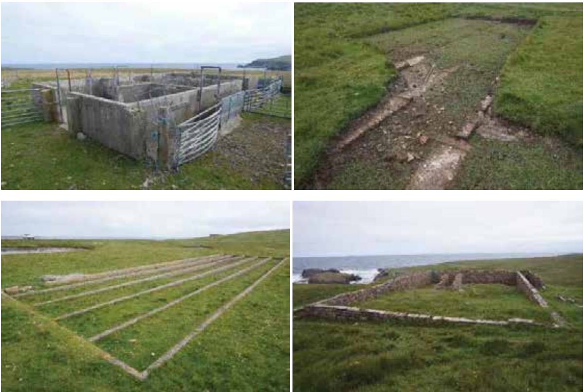
Figs. 7 to 10: Most ancillary structures comprise lowered brick walls, sleeper walls and concrete foundations.
