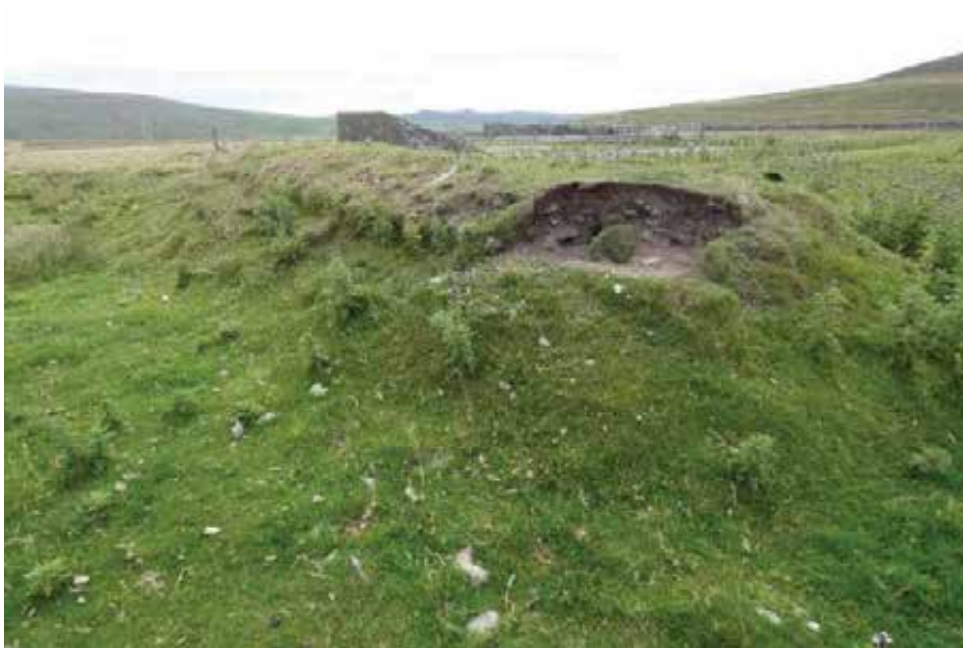
General view from southeast. Note damage caused by grazing and burrowing animals. Replacing the missing and damaged earth and turf banking will protect the structure below.
