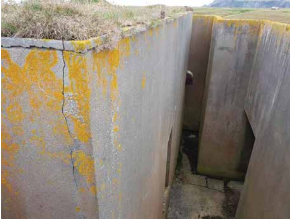
Looking down into the perimeter walkway between blast walls and building.
