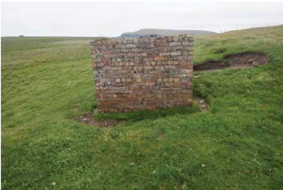
No structural cracking was observed despite the walls not being plumb or level.
