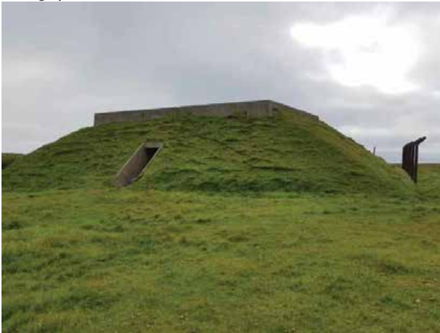
General view of the structure. The embankment is laid against RC blast walls about the building itself.
