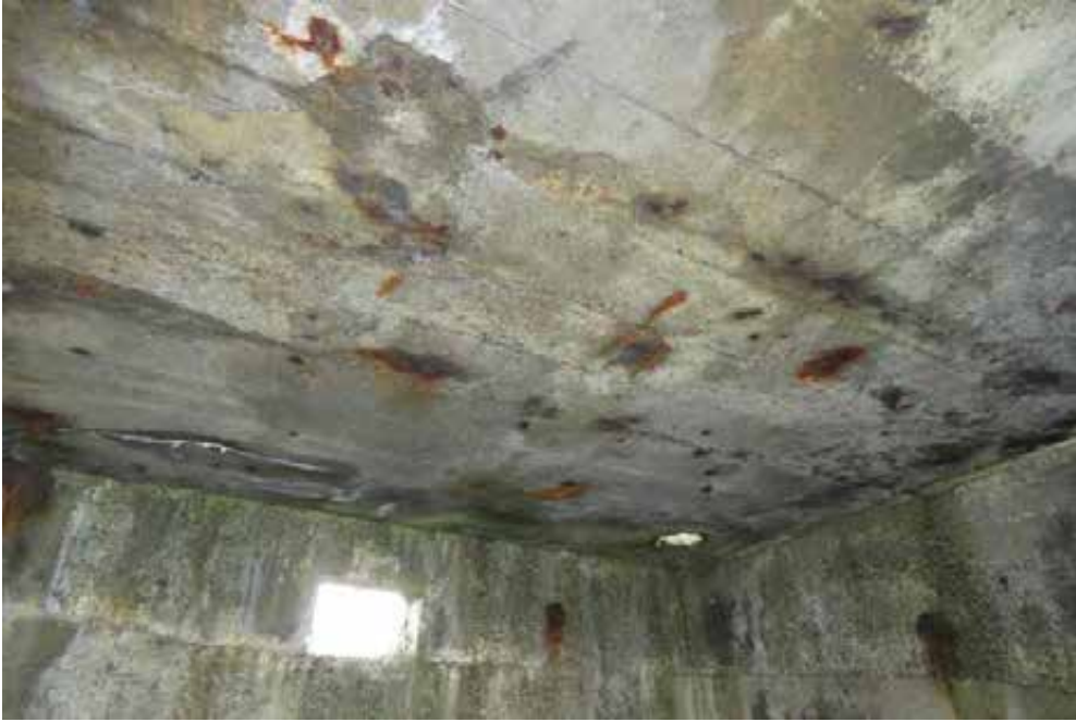
Hairline cracking, rust staining, leaching and discolouration to the soffit of the roof structure.
