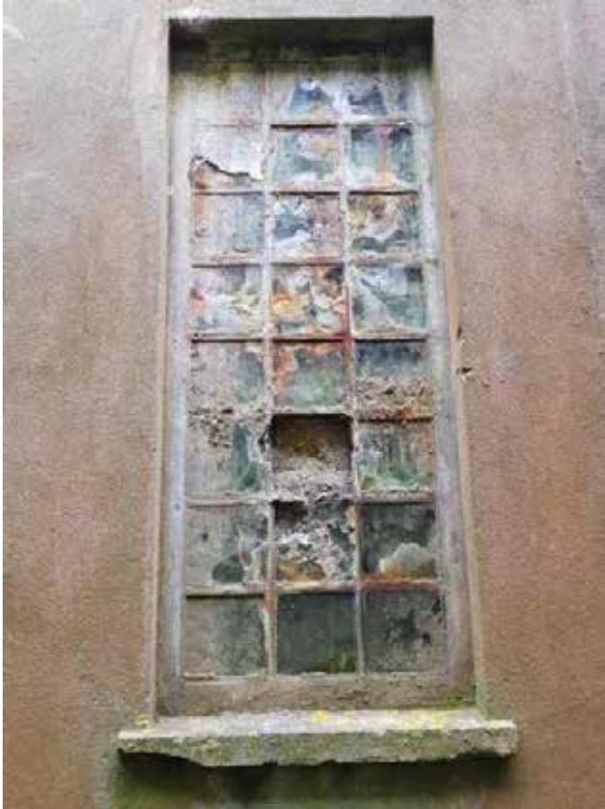
A surviving window frame.
