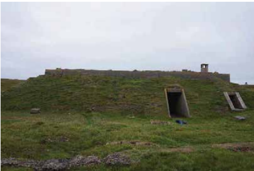
Fig. 2a & 2b: Blast walls were constructed of reinforced concrete, cast in situ, with sloping earth banks externally to protect for the brick and concrete operational buildings of the Chain Home.
