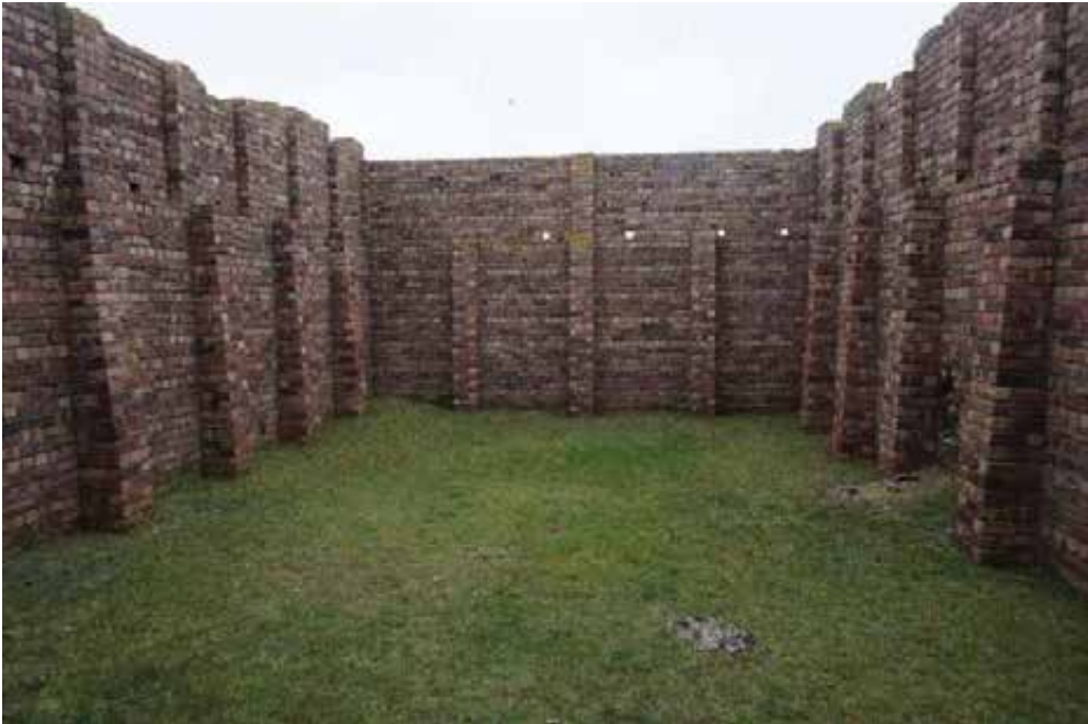
Internal general view.
