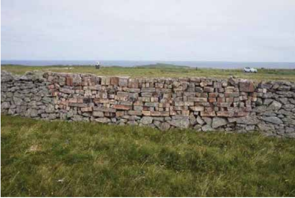
The repair using salvaged bricks c.40m north of the access road remains in good condition.
