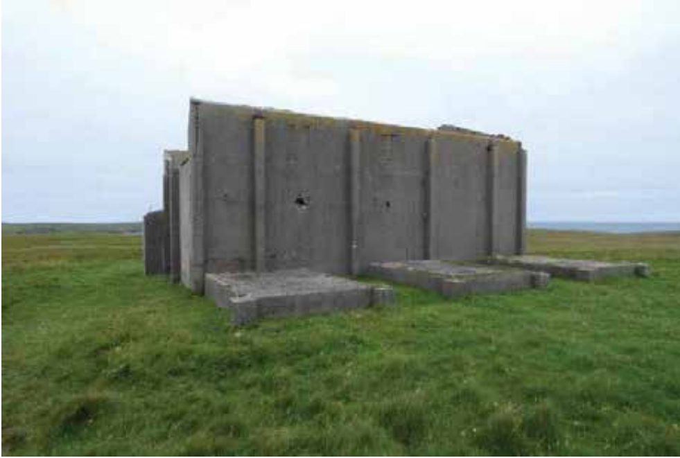
South elevation. See photos 2 and 4. This wall is a tall, thin, free-standing element.
