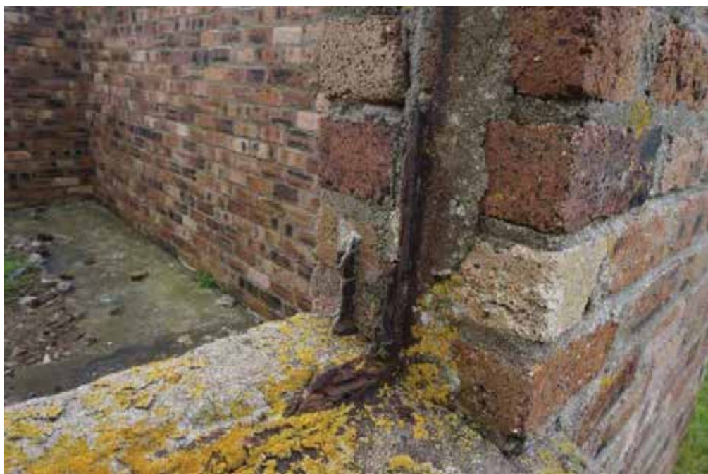
Evidence for metal window frames survives within window checks.
