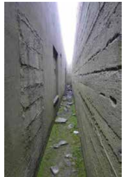
Fig. 2a & 2b: Blast walls were constructed of reinforced concrete, cast in situ, with sloping earth banks externally to protect for the brick and concrete operational buildings of the Chain Home.
