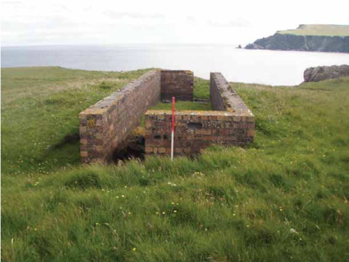
Plate 62: South-east facing view of probable air raid shelter (Site 105)
