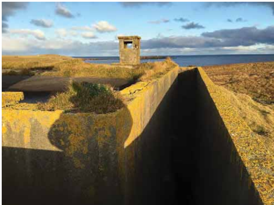
Large Bunker roof and external walls (typical)
