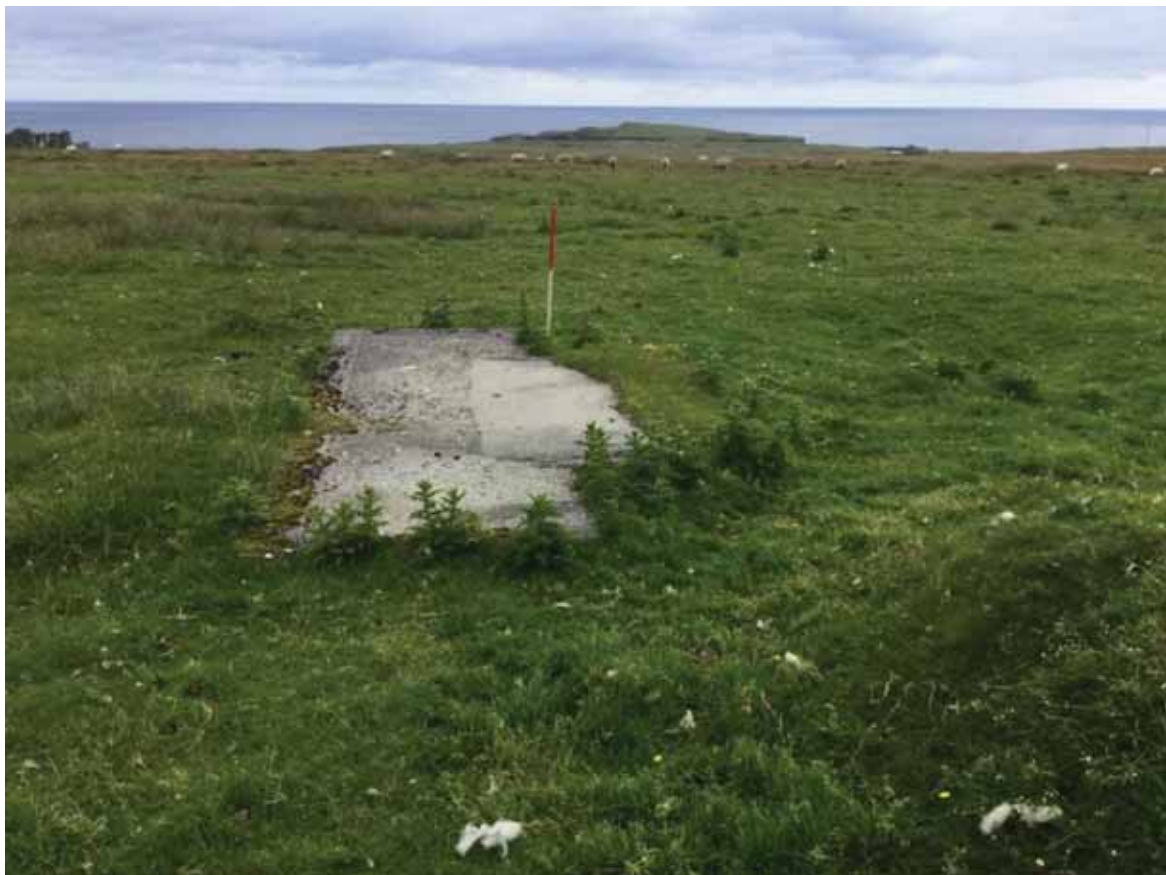
Plate 24: East facing view of a concrete foundation (Site 307)
