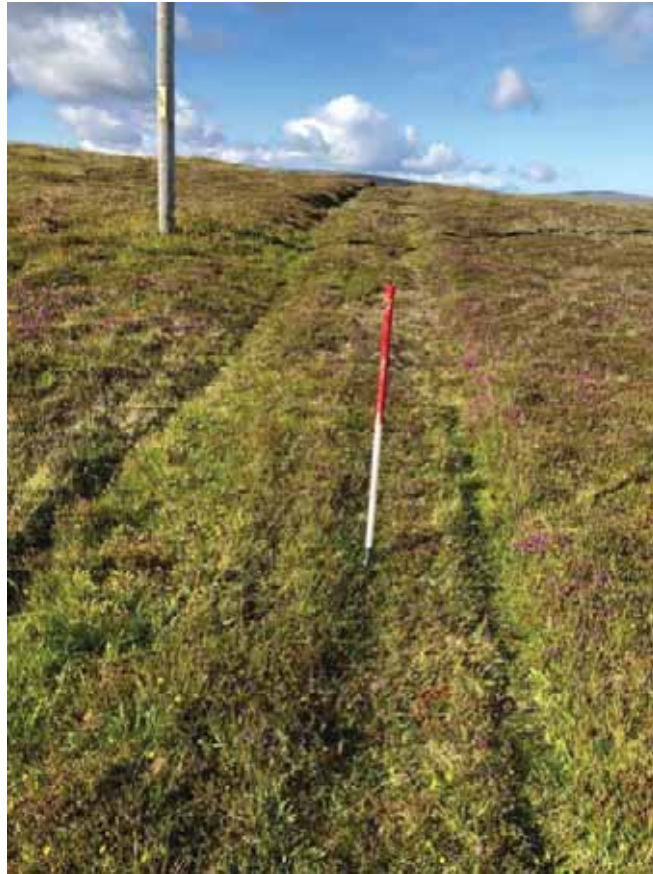
Plate 139: South-west facing view of the New Section of Access Road
