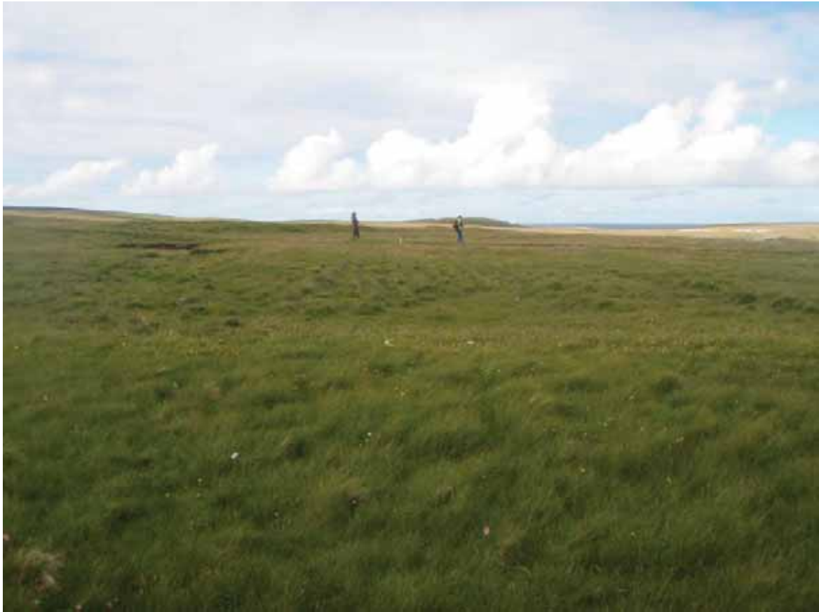
Plate 65: North facing view of the overgrown remains of a billet block (Site 106)
