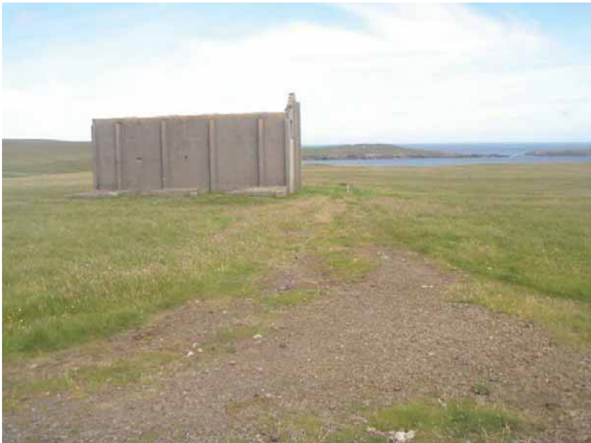
Plate 52: North facing view of the power house (Site 77), with its three concrete platforms and the northwards extending track (Site 77d)
