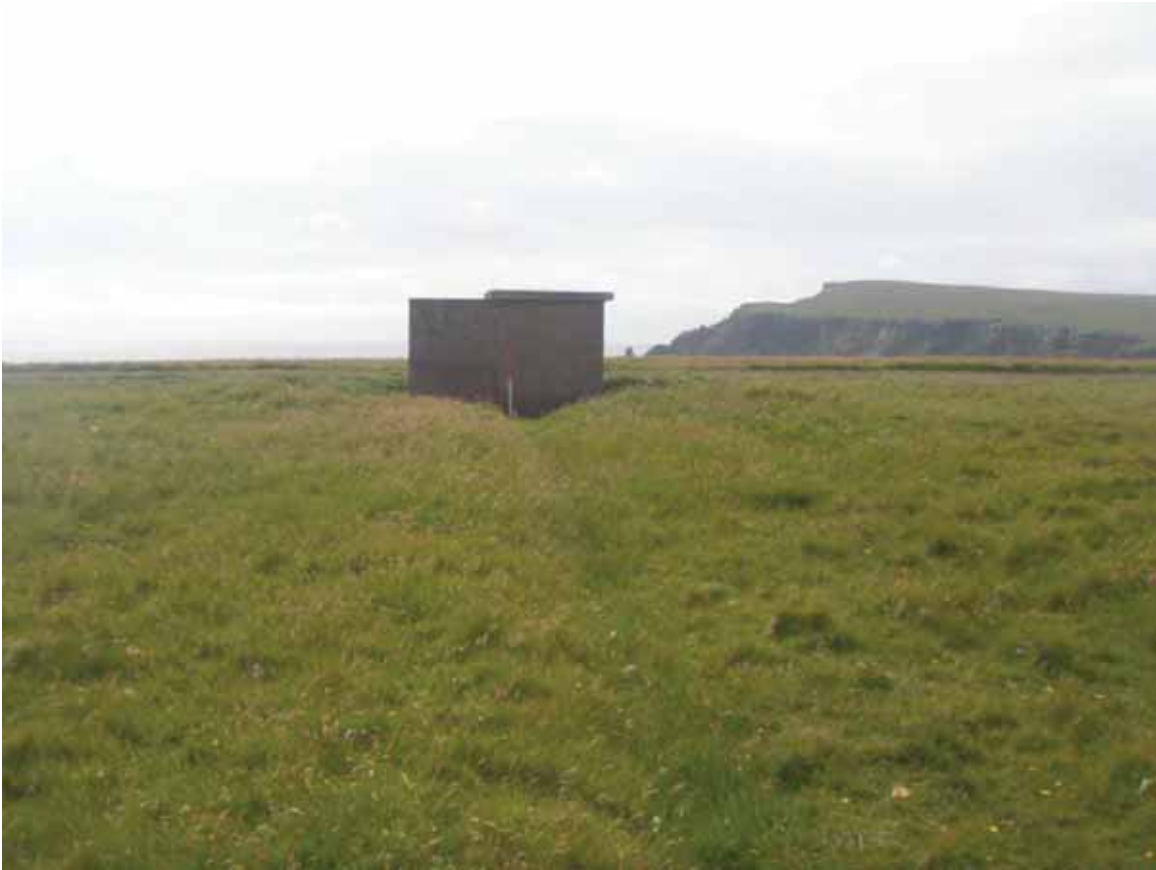
Plate 57: South facing view of channel, potentially a service channel to the north of the guard hut (Site 82)
