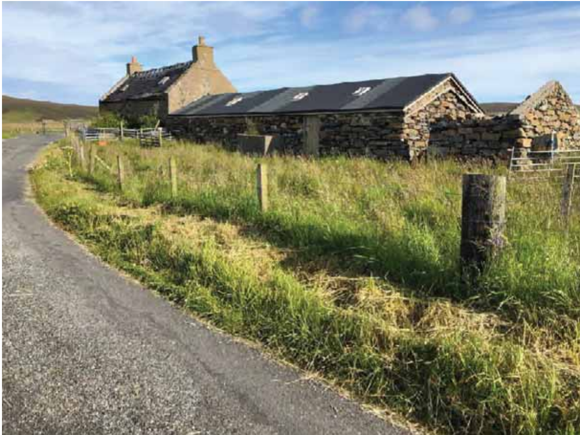
Plate 147: North-west facing view of the Category B Listed Papil (Site 5)
