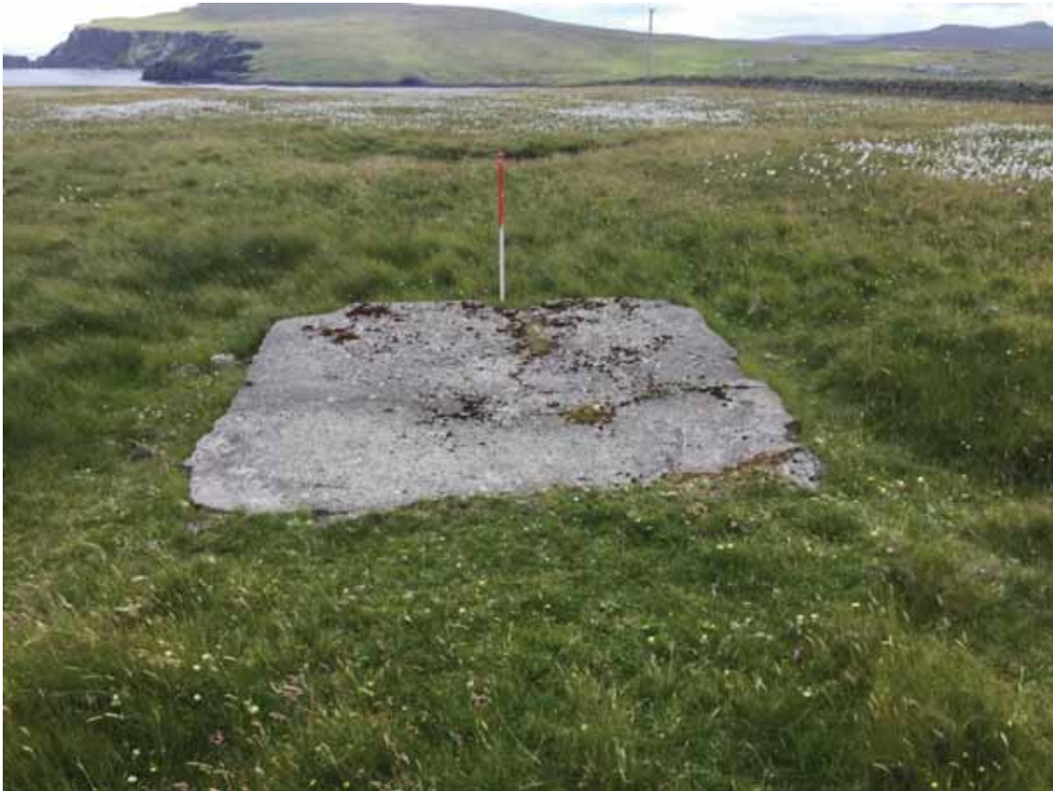
Plate 21: South facing view of concrete foundation block (Site 205)
