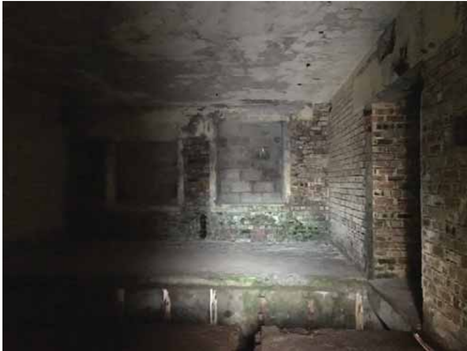
Large bunker internal (typical)
