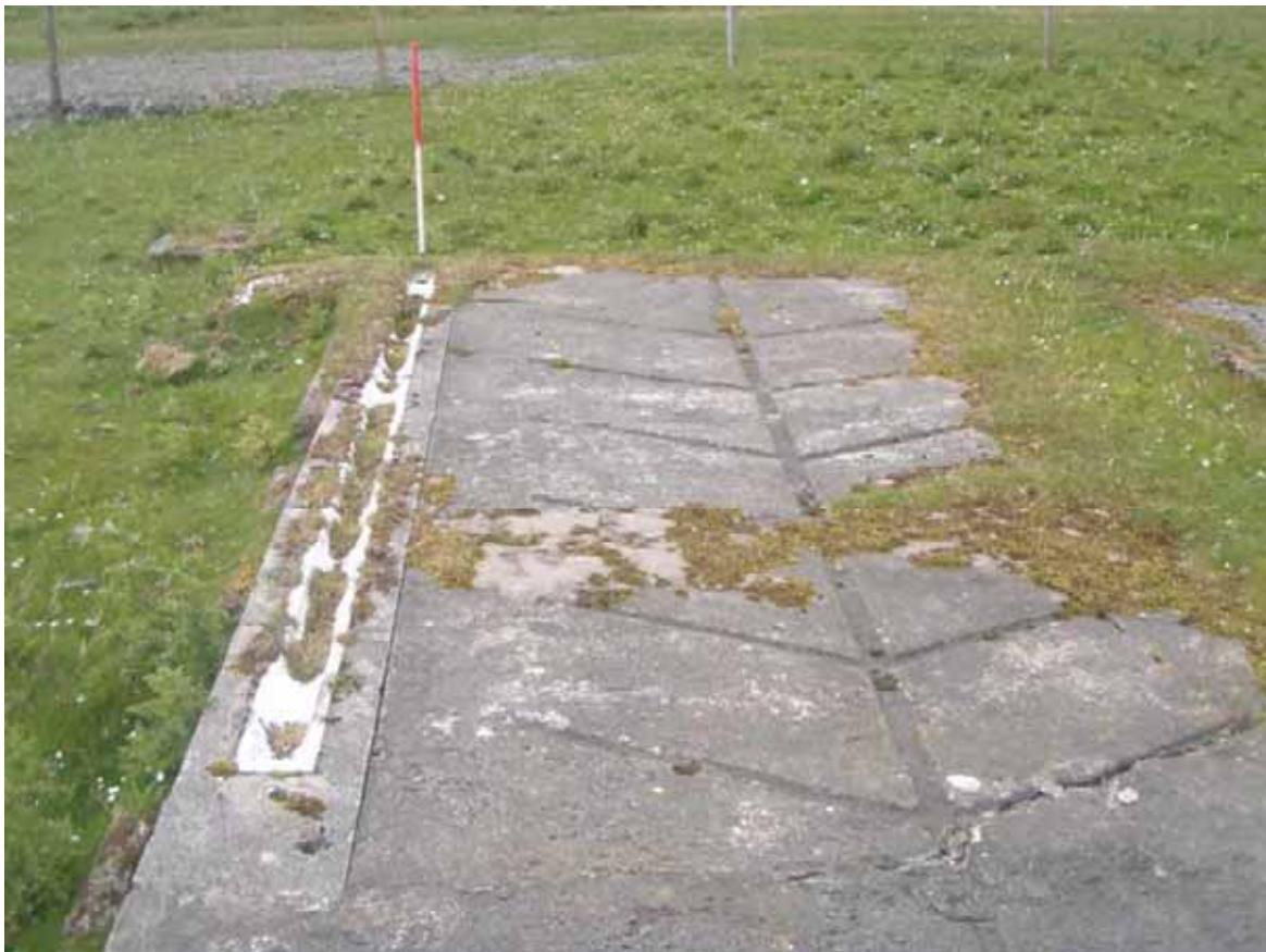
Plate 30: Detail of the remains of drainage features at the northern end of the abultions block (Site 132)
