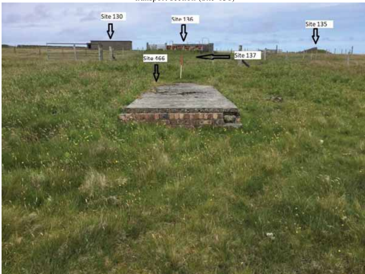
Plate 34: Northing facing view of the concrete capped brick structure (Site 446)
