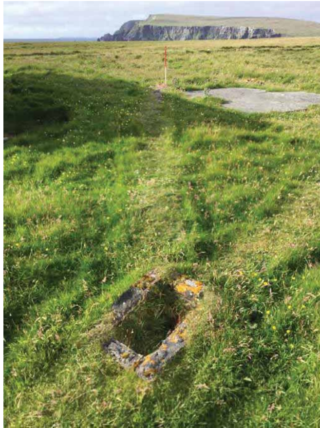
Plate 75: South facing view of a pipe (Site 428) on the eastern side of a concrete pad (Site 84b). The pipes (Site 427 & 428) converge at a brick structure in the foreground
