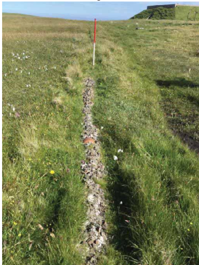
Plate 100: South-east facing view of pipe (Site 411) which may connect to the probable toilets (Sites 412-4)
