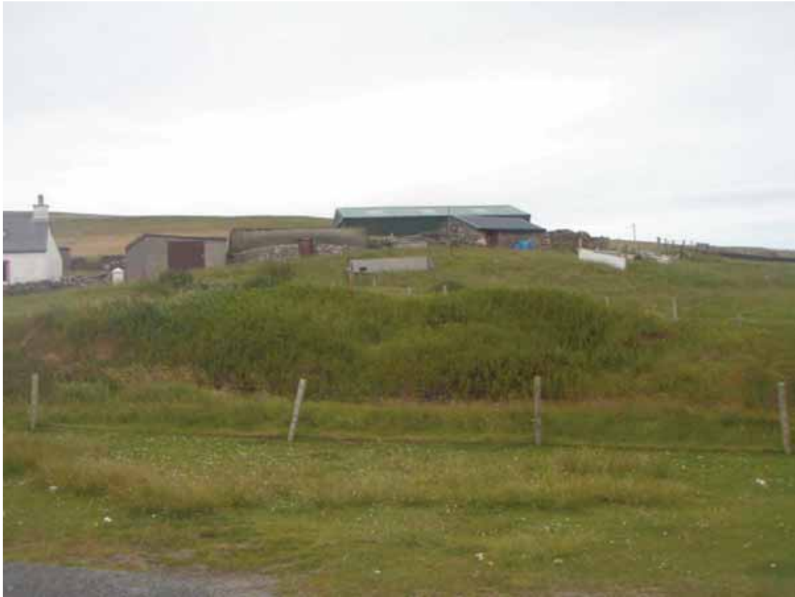
Plate 149: North facing view of the Category C Listed Boat-roofed shed (Site 6)
