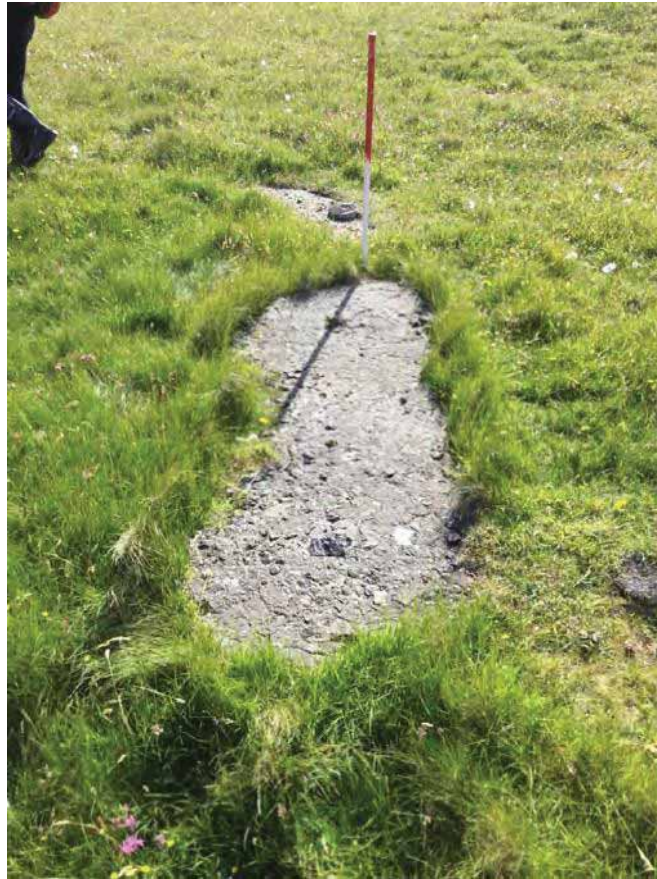
Plate 137: Detail of concrete block (Site 405)
