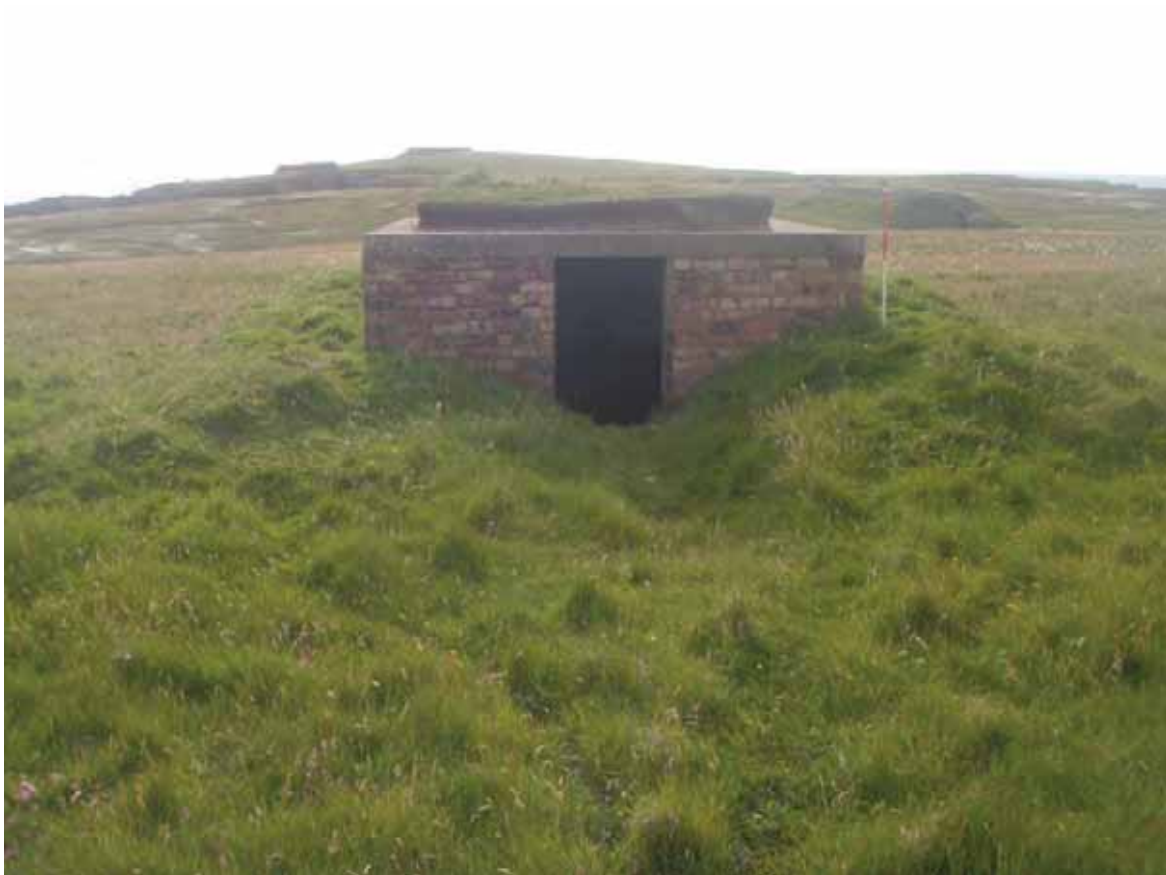
Plate 94: East facing view of a potential air raid shelter (Site 87)
