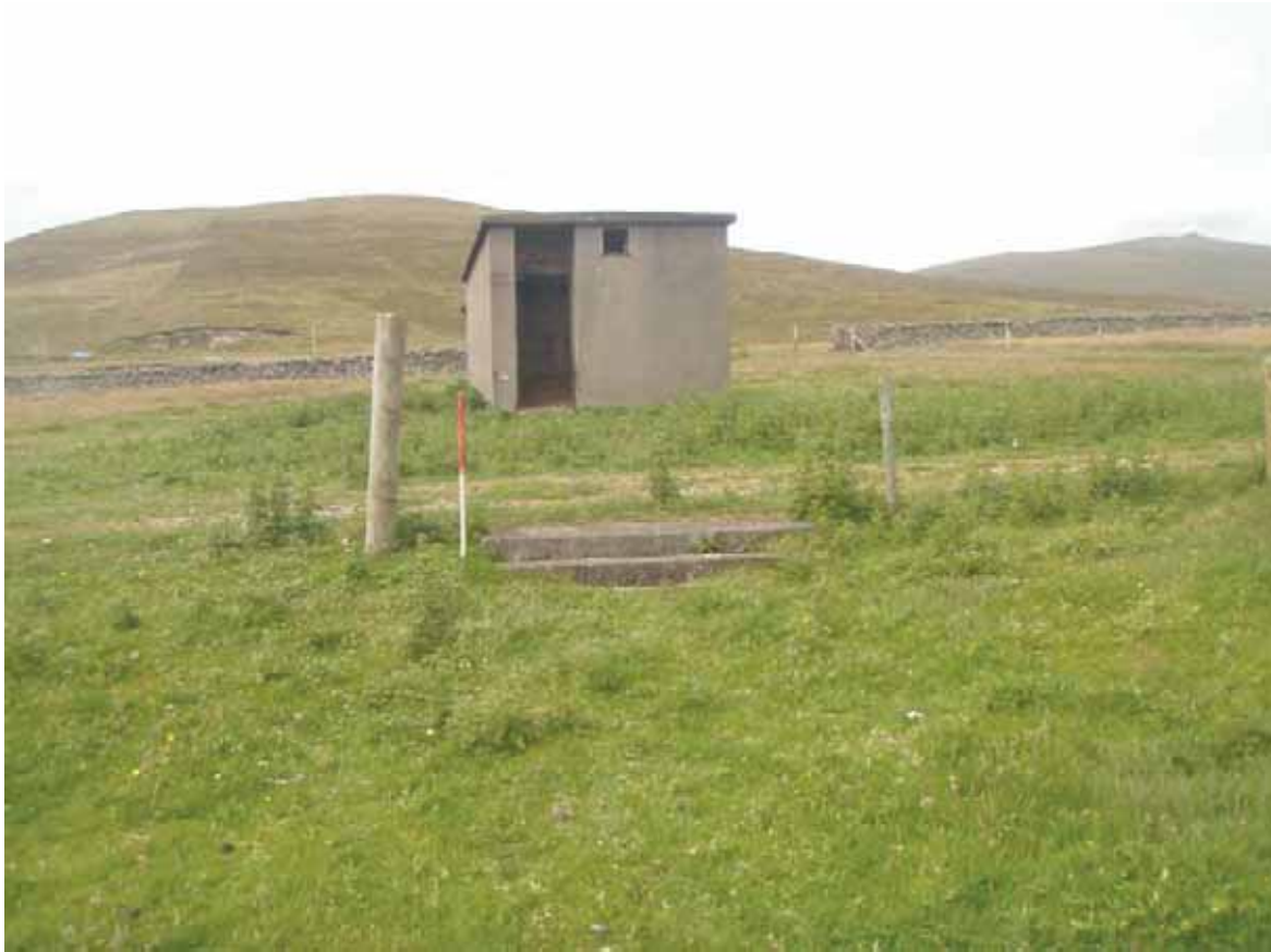
Plate 25: West facing view of the steps between the decontamination block (Site 130) and the former air raid shelter (Site 134)
