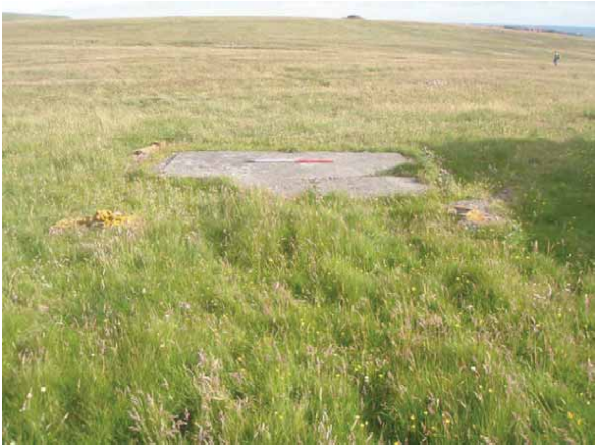
Plate 73: North facing view of concrete pad (Site 84b) with a concrete pipe (Site 428), originating from the south-east corner, visible
