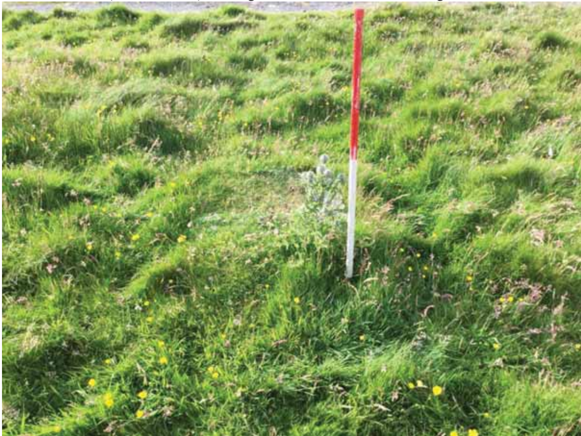
Plate 76: South facing detail of an overgrown concrete base (Site 426)
