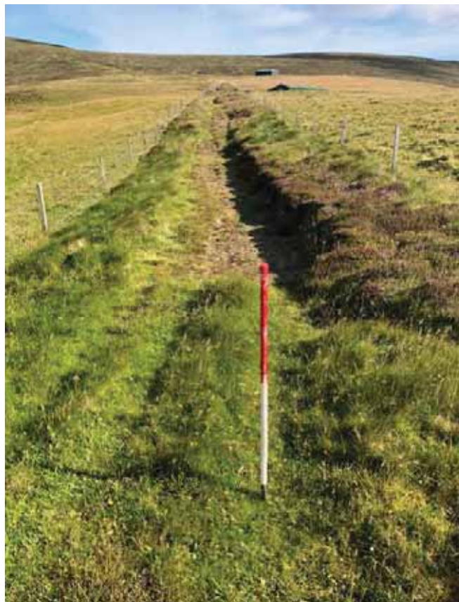
Plate 140: Northing facing view of New Section of Access Road
