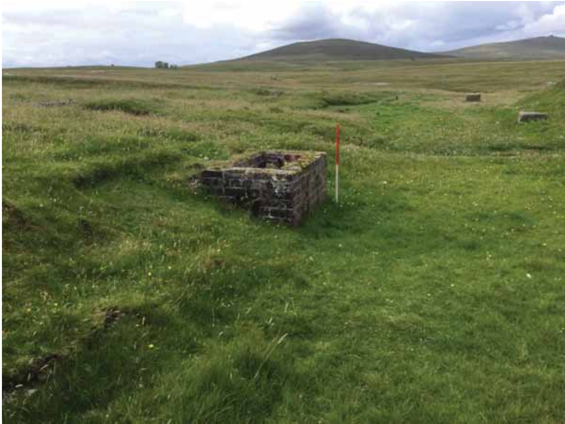
Plate 83: West facing view of a brick structure (Site 302) within the area encircled by Site 85b
