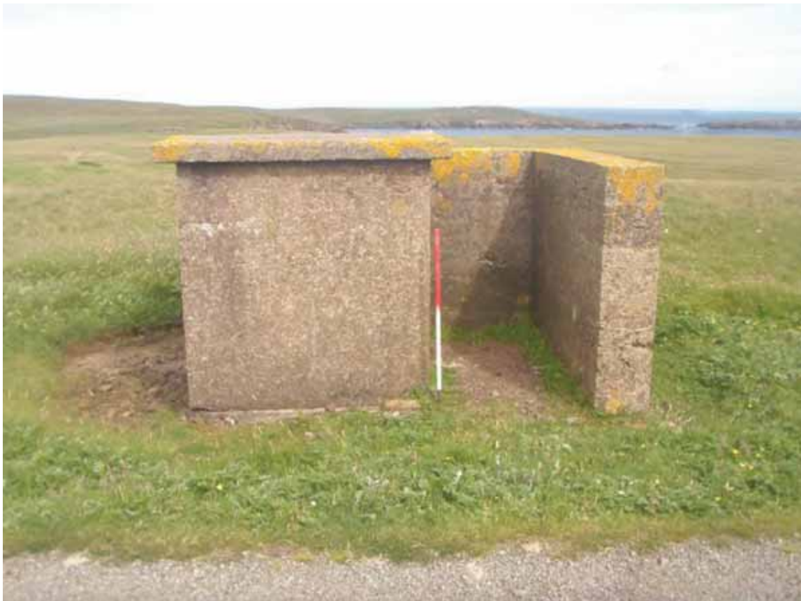
Plate 56: North facing view of guard hut (Site 82)
