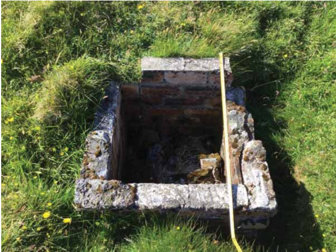
Plate 77: Detail of brick structure (Site 378)
