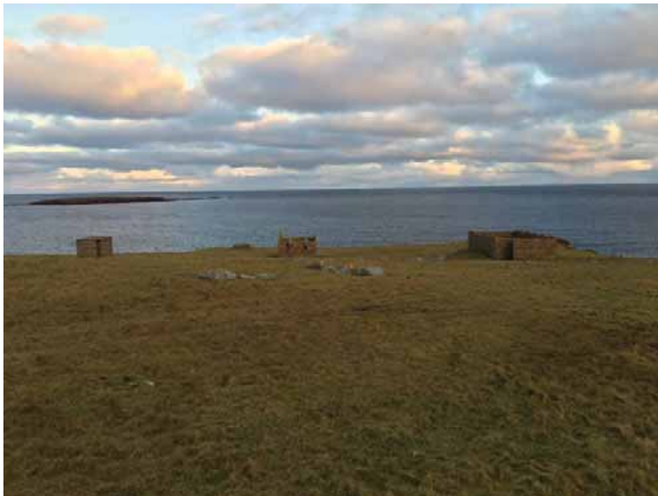
Typical Small Buildings
