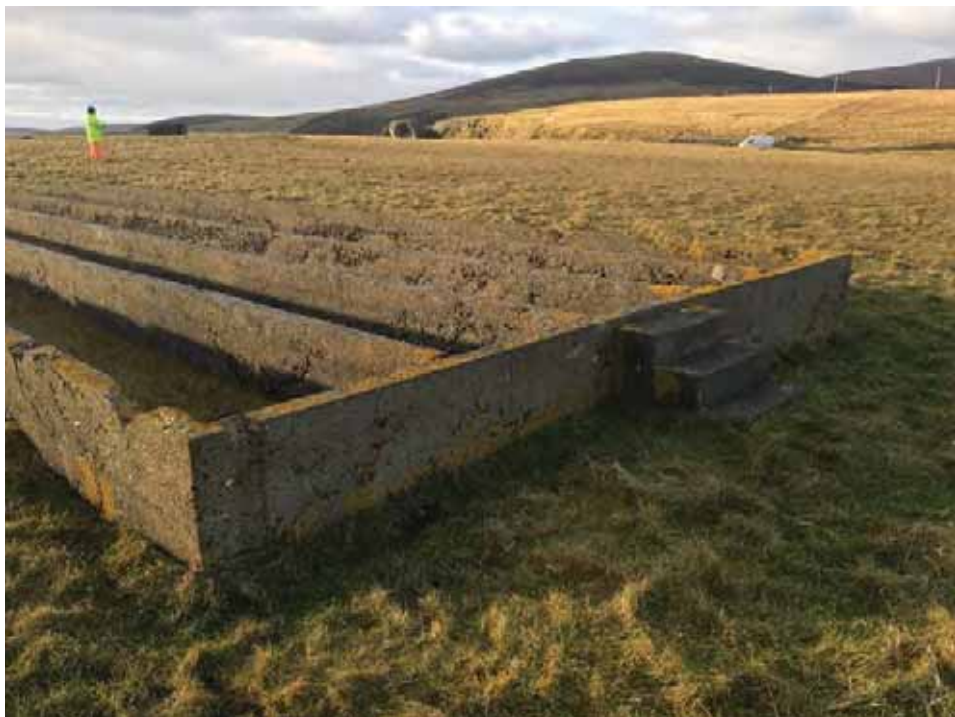
Former building foundations
