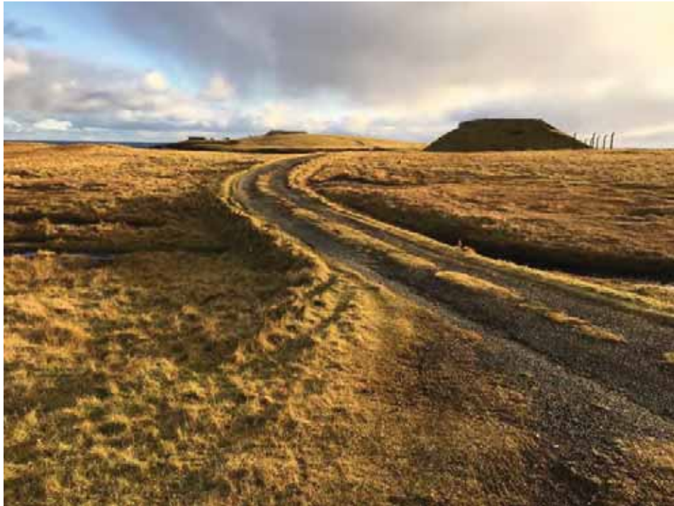
Typical existing road condition
