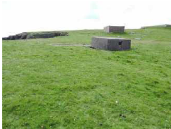
Photo 4. Reverse view from proposed hide location, looking back inland towards existing old RAF buildings, 2020.
